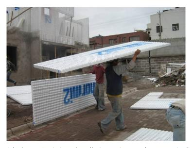
The lighter the material, the easier it is to handle it on site. Furthermore, its lightweight makes it possible to reduce and in some cases even avoid the use of mechanical means which are also energy consumers and therefore also producers of climate-altering substances.
